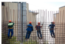
Iron bars for building construction
